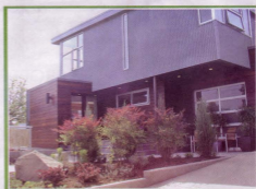
The house at 169 Lynn St. in its new incarnation. The project was undertaken by Rob and Stephanie deGaetano's company, redesign.
